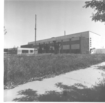
Radioactive waste processing
